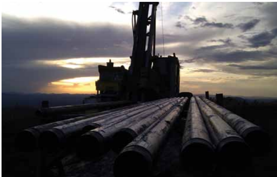
At the end of the day, the company is hoping to become a multi-niche metal producer.
